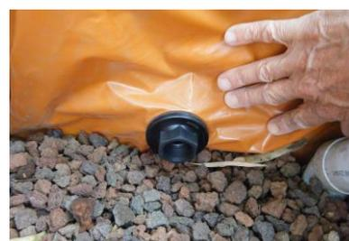
5 – tank fitting placed through plastic lining and bed wall
